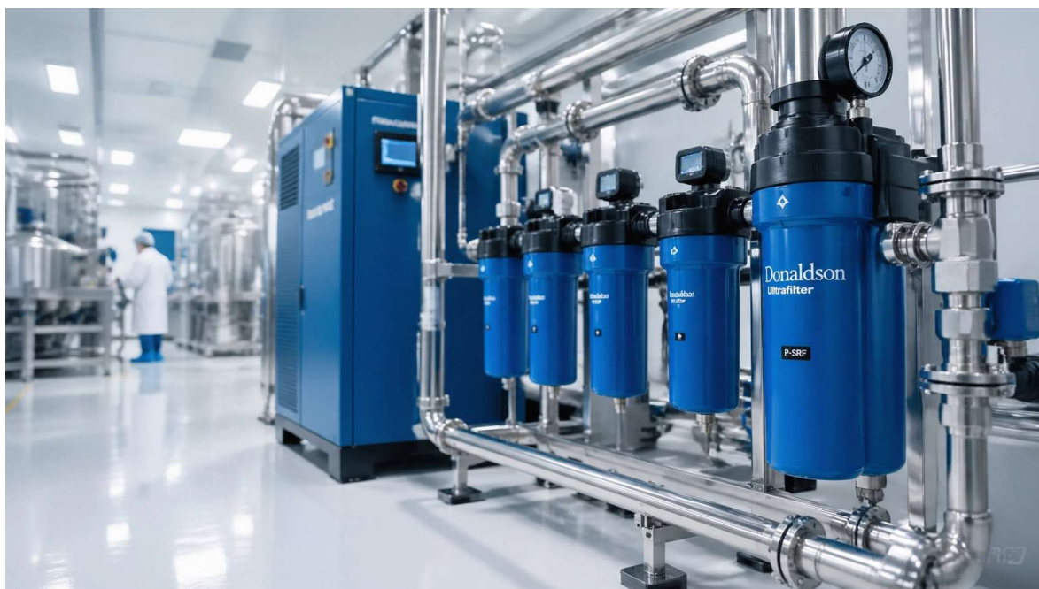
Caption: High-efficiency filtration modules used in tandem with oil-free systems to maintain ISO Class 0 standards.
